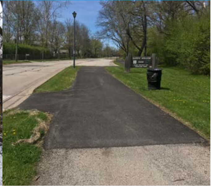
Trail extension on Trail Way
